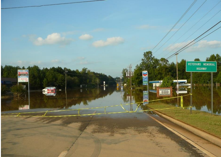
Figure 3: 2009 Sweetwater Creek flooding at Veterans Memorial Highway
